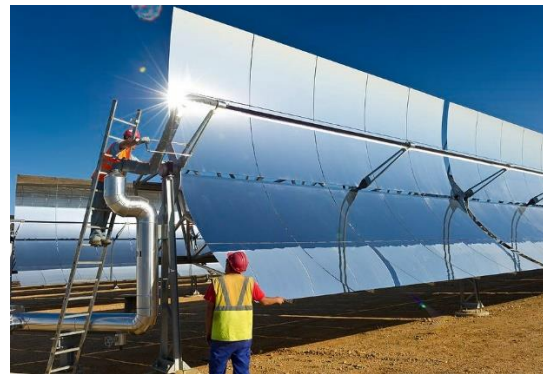
Figura 3.4 – Parabolic Trough Solar Power Plant [21].
