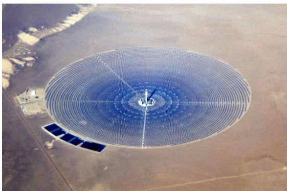
Figura 3.5 – Torre de Energia Solar situada Nye County School District, NV, USA [22].
