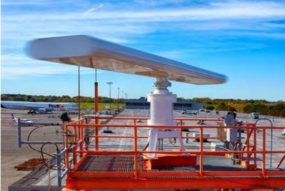
Figure 8. Air Traffic Control ASDE-X Ground Radar Unit (Source: SAAB)
