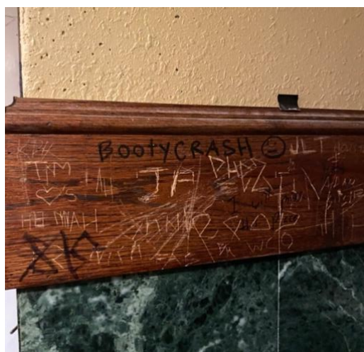
Figure 1: Segment of DSP Bathroom.
