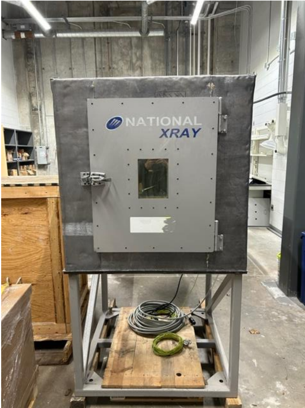
Figure 26. Finished X-ray cabinet with the door mounted and all shielding requirements met.
