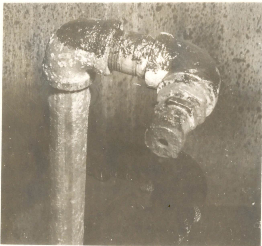
Figure 13. Filter Flow Control Orifice.
