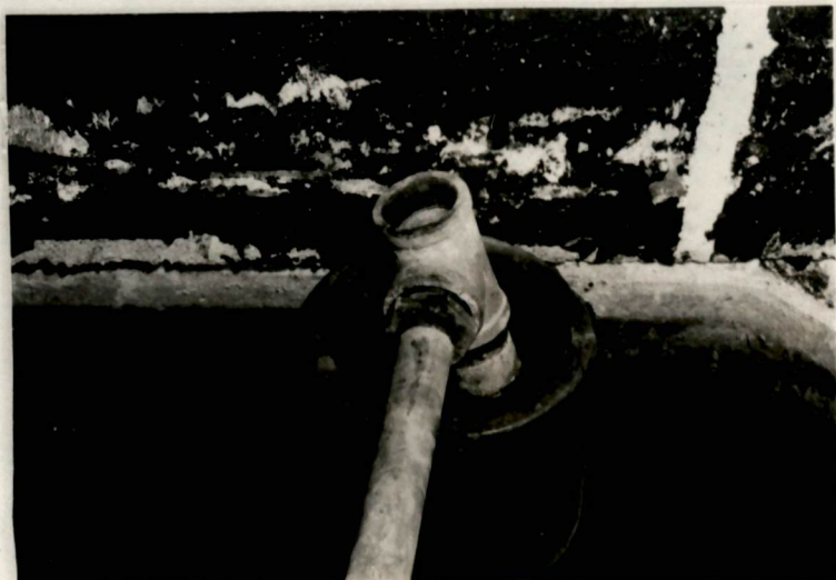
Figure 10. Six-inch Bell Tile Coagulant Mixer.
