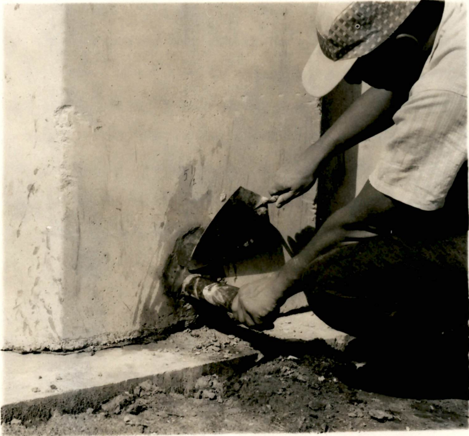
Figure 11. Method of Installing Pipes in Tanks.
