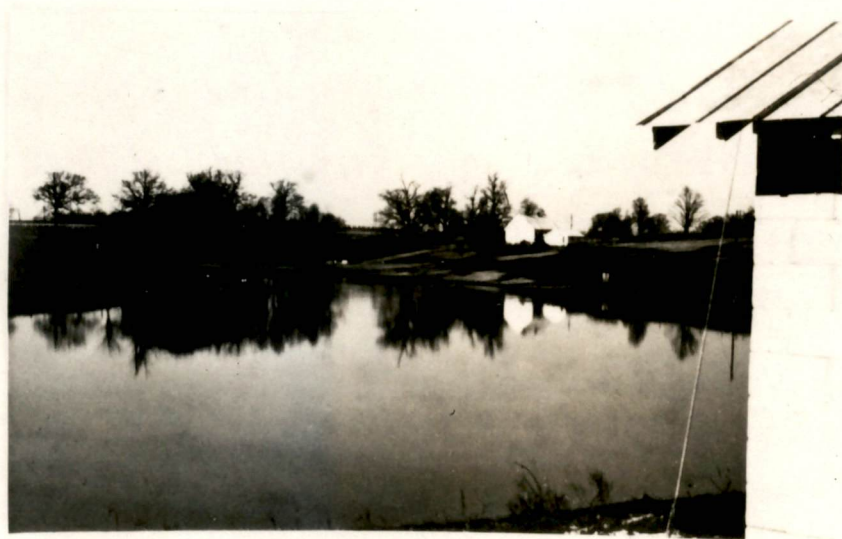
Figure 3. View of 8.6 Acre Pond Facing Away From Dam
