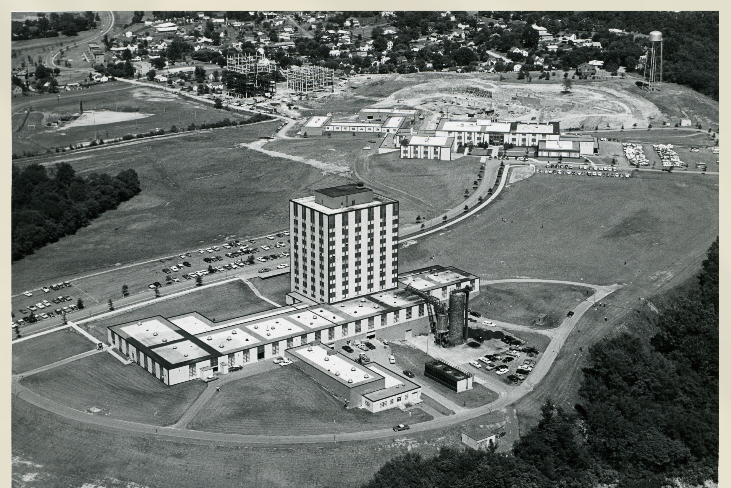
Evansdale campus, 1965, including Engineering building and early construction of Towers Residential Complex with Evansdale neighborhood in the background. Credit: West Virginia University and Regional History Center, WVU Libraries
