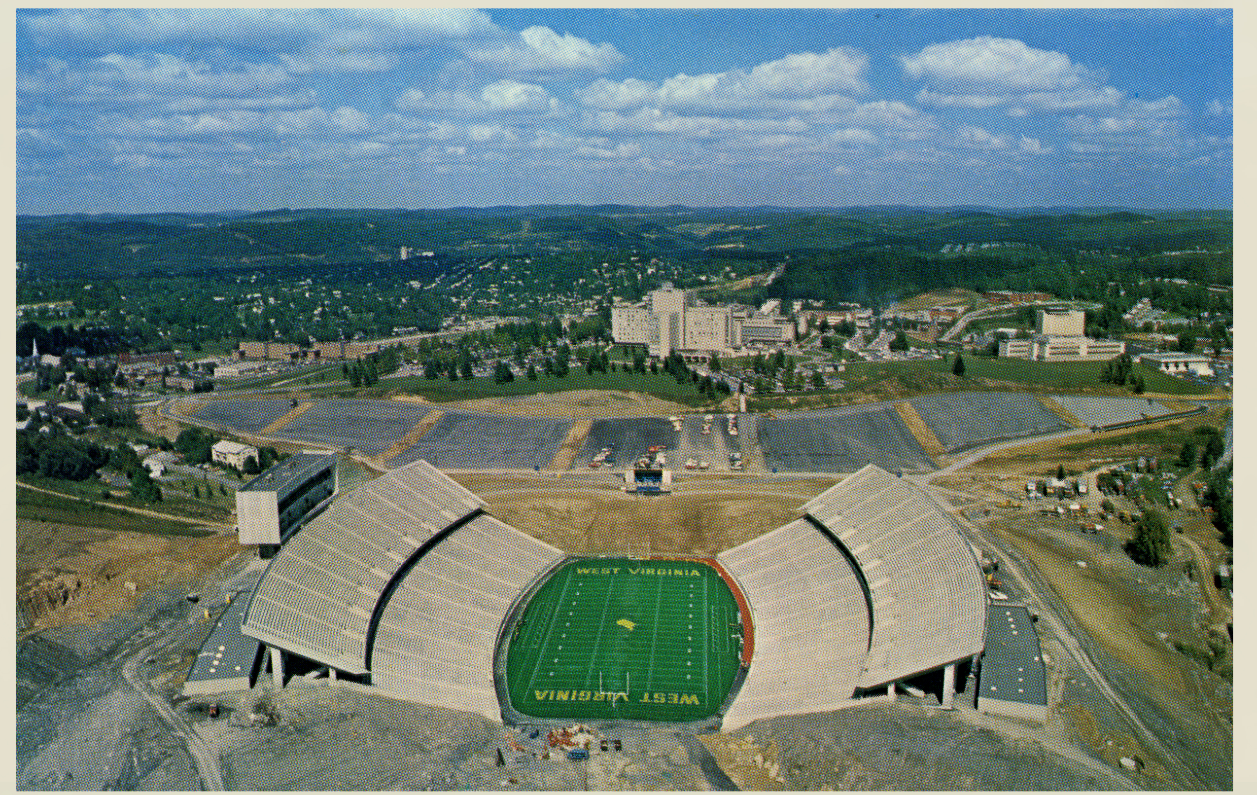
Construction of the new Mountaineer Field, circa 1980. Credit: West Virginia University and Regional History Center, WVU Libraries
