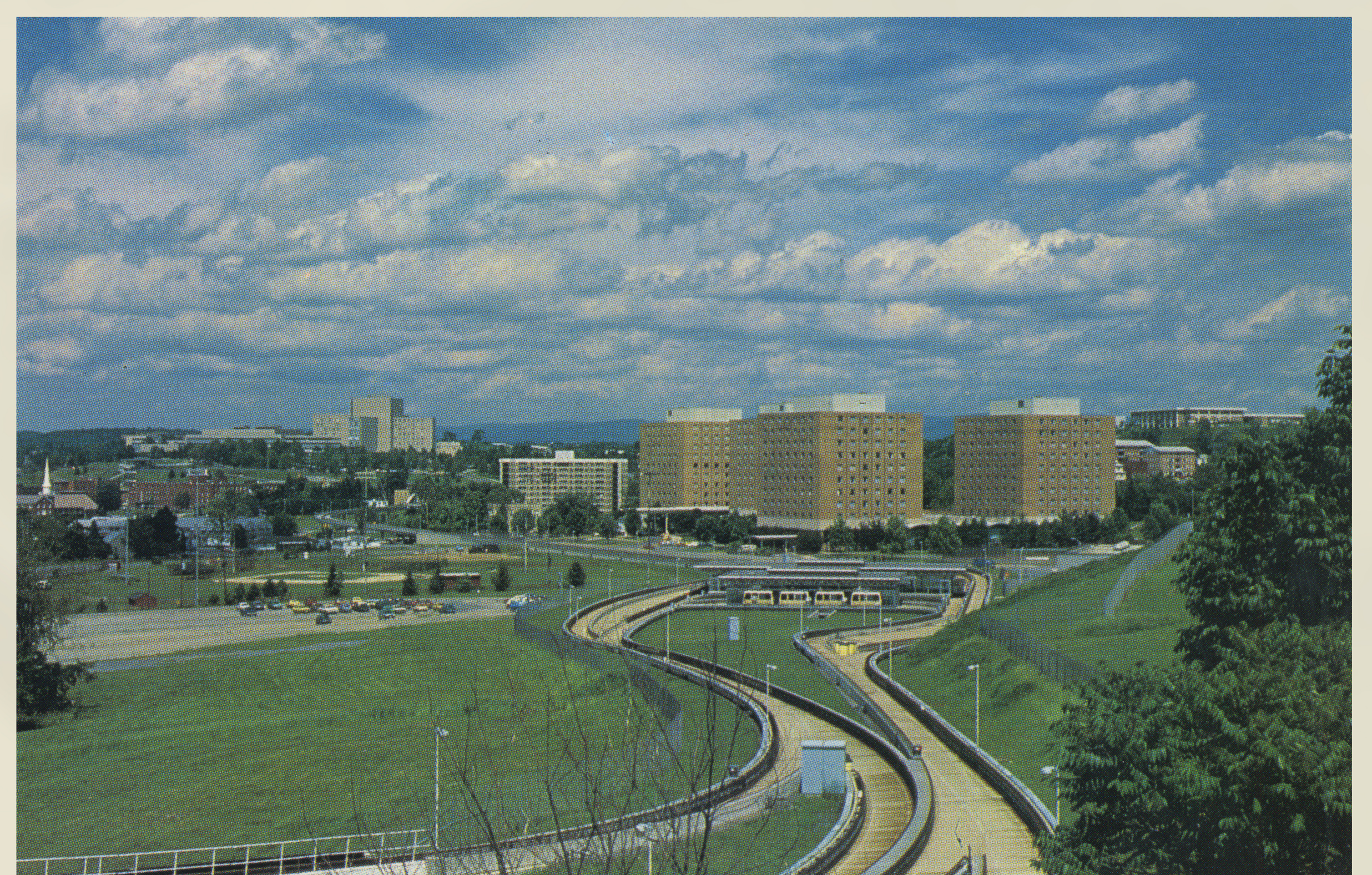
View of Evansdale campus after construction of the PRT. Credit: West Virginia University and Regional History Center, WVU Libraries
