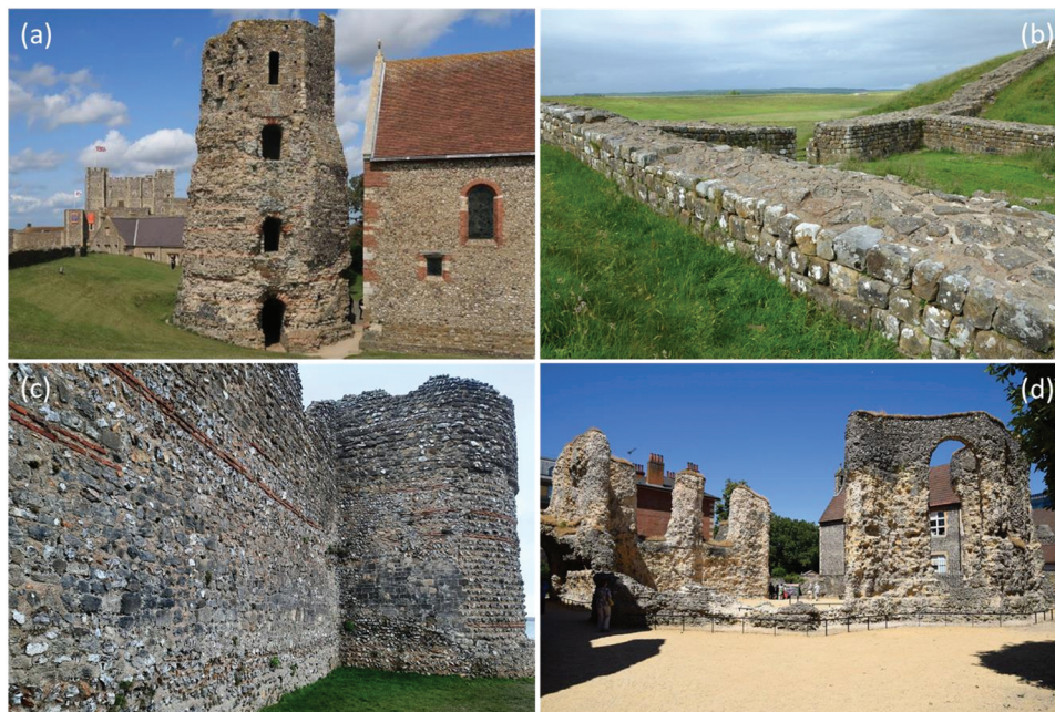
Figure 6. Early concrete in Britain. (a) the Roman 'Pharos' Lighthouse [Alexander Kachkaev 2012, CC BY-SA 3.0]. (b) Hadrian's Wall [Carole Raddato 2017, CC BY-SA 2.0]. (c) the exterior walls of Portchester Castle [Jamie Heath 2021 CC BY-SA 2]. (d) Remains of the concrete core of Reading Abbey [Hugh Llewelyn 2018, CC BY-SA 2.0].
