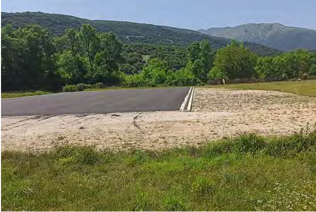
Figure 8: Half-finished football pitch; picture taken by KA2
