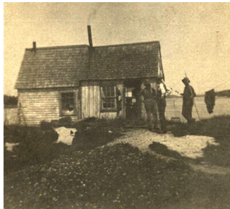
House on Malaga [Courtesy of Peter K. Roberts]
