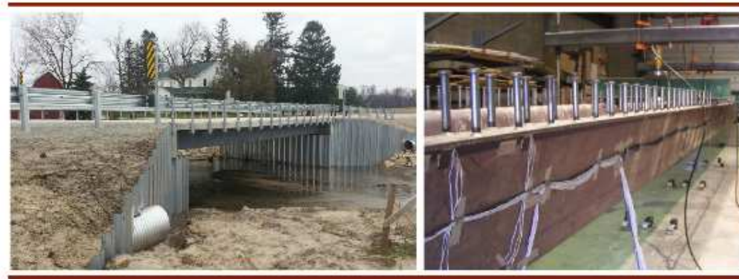
Figura 1: Puente Amish Sawmill, extraída de Evaluation of a Folded Plate Girder Bridge System Final Report June 2017
