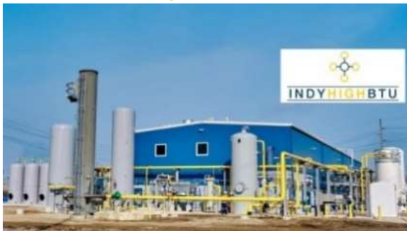
Indy HBTU Plant
