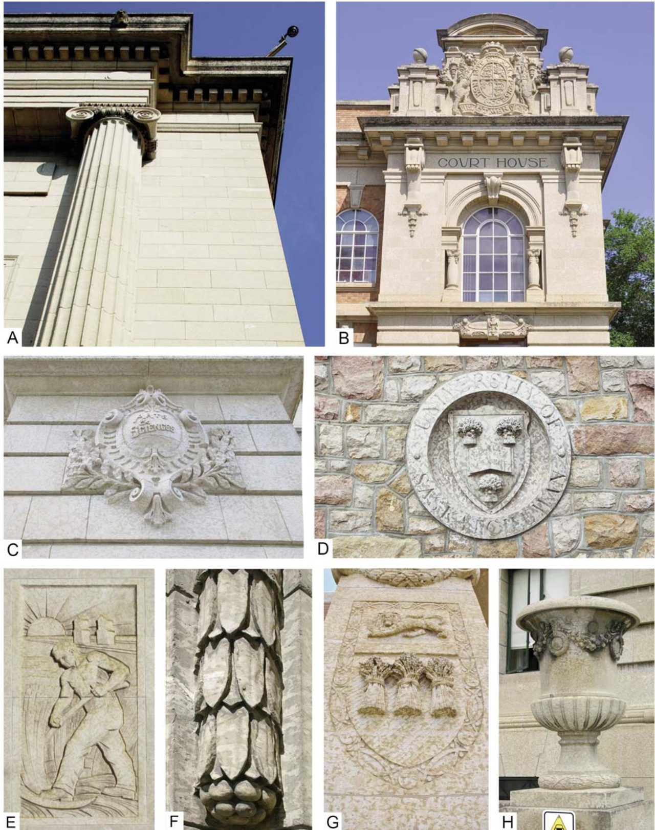
Figure 21. Examples of carved Tyndall stone. A. Fluted column with Ionic capital. Manitoba Legislative Building. B. Façade with pediment, various ornaments and coat of arms of the United Kingdom. Courthouse, Humboldt, Saskatchewan. C. Ornamental element with laurel wreath in honour of the arts and sciences. Carnegie Library, Winnipeg. D. Crest of the University of Saskatchewan. E. Sculpture of farm worker scything with grain elevators and rising sun behind. Bank of Montreal Building, Saskatoon (also Figure 29E). F. Ornament in the shape of tiers of leaves. Manitoba Legislative Building. G. Crest of the Province of Saskatchewan, courthouse, Battleford. H. Ornamental urn. Manitoba Legislative Building.
