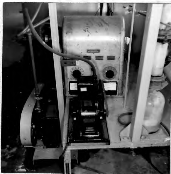
Fig. 3 - Vacuum Pumps & Furnace
