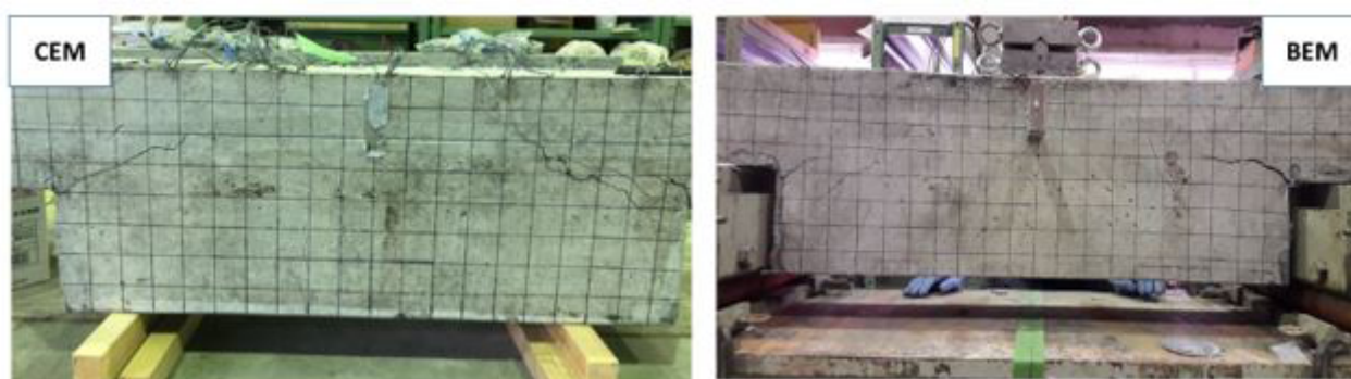
FIGURE 19. Failure pattern of RCDEB loaded at the midpoint (17).
