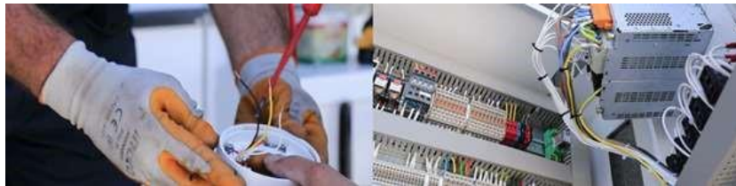
Fig.6. Photo during SCADA system installation [6]
