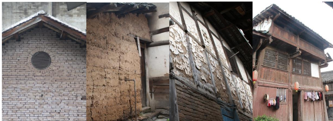
Figure 3. The Form of Enclosure Structure of Residential Houses in Enyang Ancient Town
