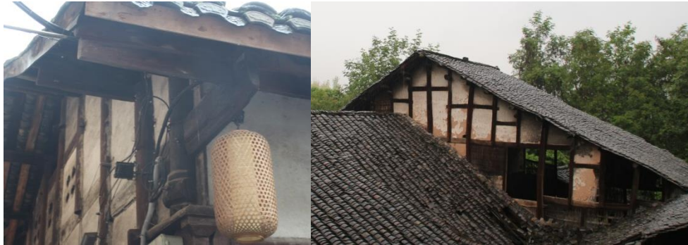
Figure 2. The Column and Tie Construction
