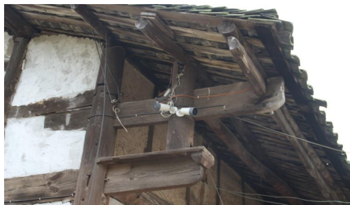
Figure 8. Triangular Stabilized Structure under the Eaves
