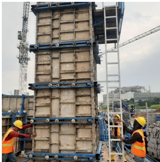
Gambar 2 Bekisting Konvensional dan Bekisting Aluminium
