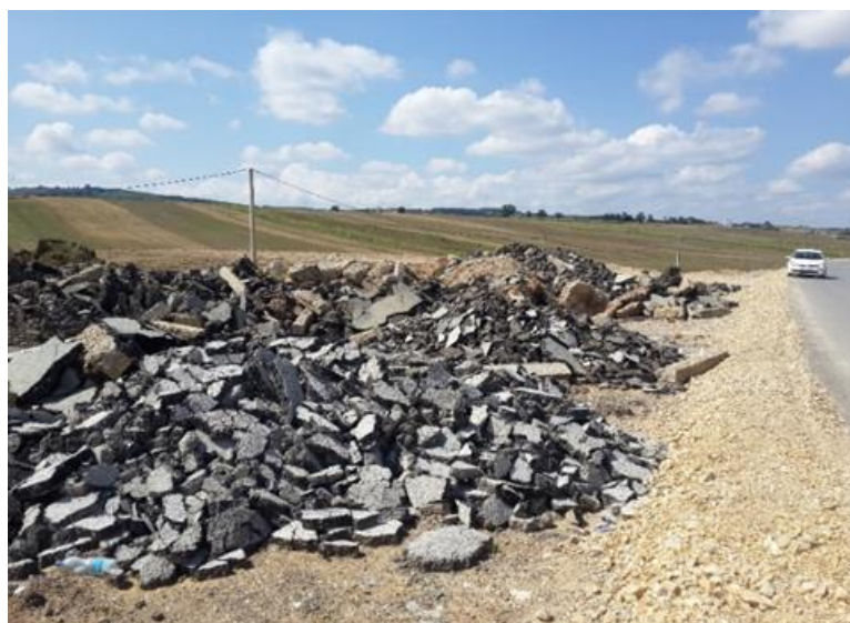
Figure 5. Full-Depth Demolition of asphalt thickness 15 to 30 cm
