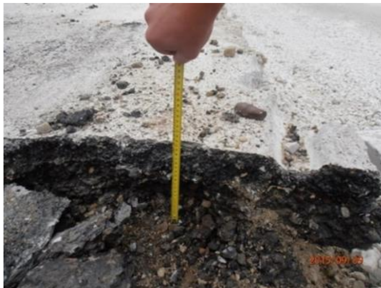
Figure 4. Full-Depth demolition of asphalt thickness 15 to 30 cm
