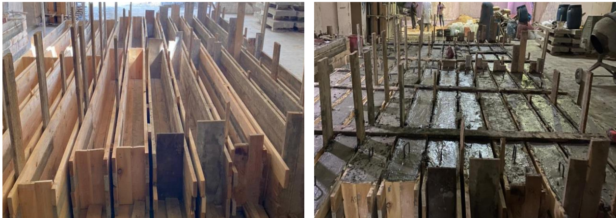
Figure 4. Fabrication process before and after casting
