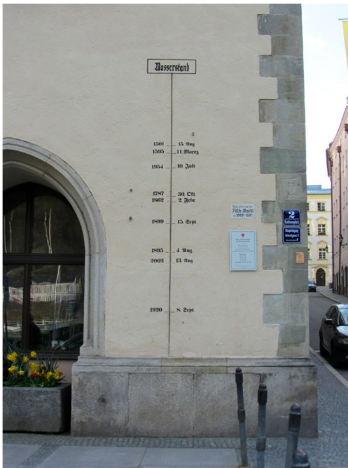
Fig. 3 Maximum water heights recorded at Passau in Lower Bavaria (Germany). The town lies at the confluence of the Danube, Inn and Ilz rivers and has regularly been flooded (courtesy of Sally Forwood)
