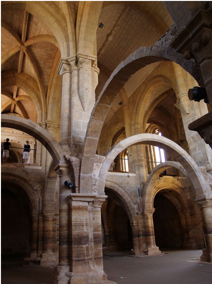
Fig. 9 The interior of the monastic church at Clara-a-Velha in Coimbra (Portugal). To escape the floods from the nearby River Mondego, the nuns raised the floor of their church and finally built an upper storey to span its full length. Once they had relocated their altars, the celebration of Mass could continue. Here, people are seen on the partially reconstructed upper storey, and the staining from high water levels is visible on the supporting columns below (picture courtesy of Alejandra Gutiérrez)
