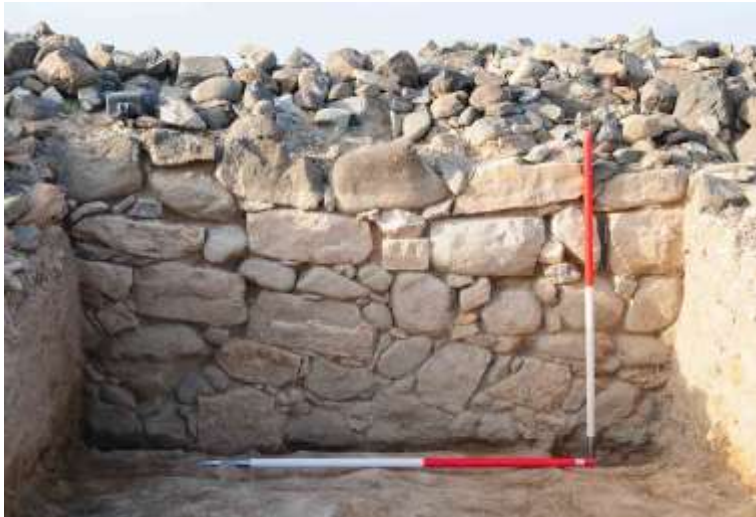
Fig. 7: View of the interior face of the main wall in Trench G showing the regular construction style.
