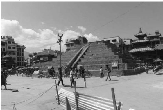
Figure 2: The foundation plinth of the collapsed Maju Degu Temple in Hanuman Dhoka's Durbar Square
