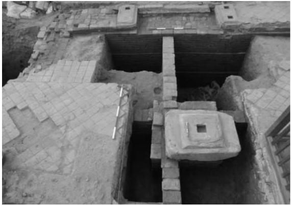
Figure 13: Saddlestone with cross-walls connecting to the brick pier.
