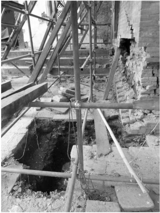
Figure 23: Unrecorded excavation trench cut alongside north facing wall of the Degutale Temple in Hanuman Dhoka's Durbar Square. Photographed in October 2015.
