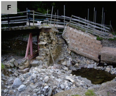
364 Fig. 3. Photographs of the impacts of Storm Desmond along St John's Beck and the surrounding floodplains. 365 (A–B) Flood sediments and debris (tree trunks) transported and deposited on floodplains and in the channel. 366 (C–D) Floodplain scour. (E) Riverbank erosion. (F) Destruction of the access bridge over St John's Beck to 367 Low Bridge End Farm (bridge approximately 3.5 m high for scale).
