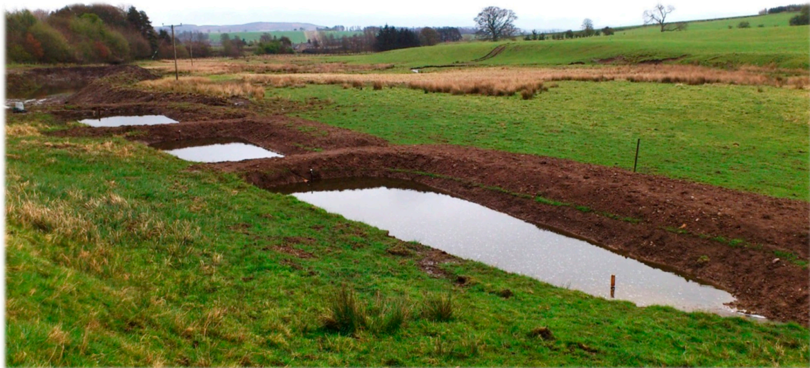
Figure 3. An example of a modified ditch with flow barriers acting as both a sediment trap and flood flow storage in Netherton Burn (photo from Barber 2013, credit to N. Barber).
