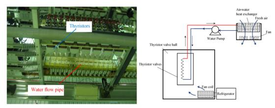
Fig. 10. Cooling system for the thyristor valves hall in Moyle.
