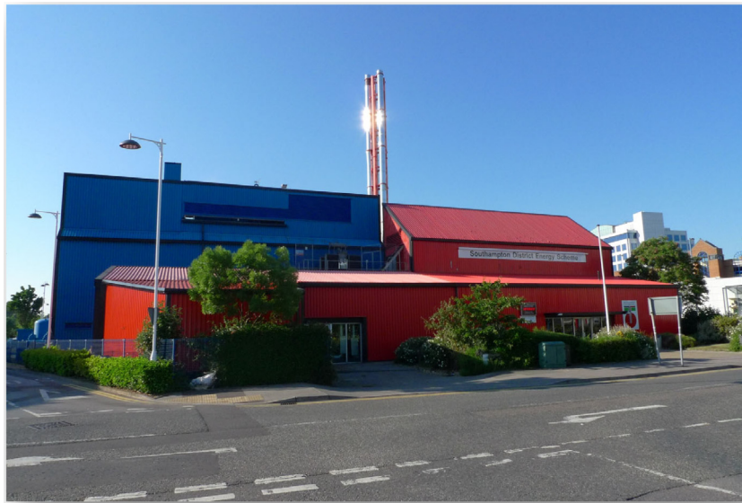
Fig. 3. Southampton District Energy Scheme operational base. The geothermal production well lies behind the building with the wellhead and associated instrumentation occupying an area of about 25 m 2 . The photograph demonstrates the modest surface footprint of a combined geothermal heat and power plant in a city centre location and absence of emissions commonly associated with a power station (photograph J. Gluyas)
