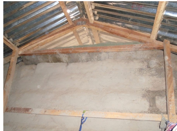
Fig. 3 RooPfs house with gable end window
