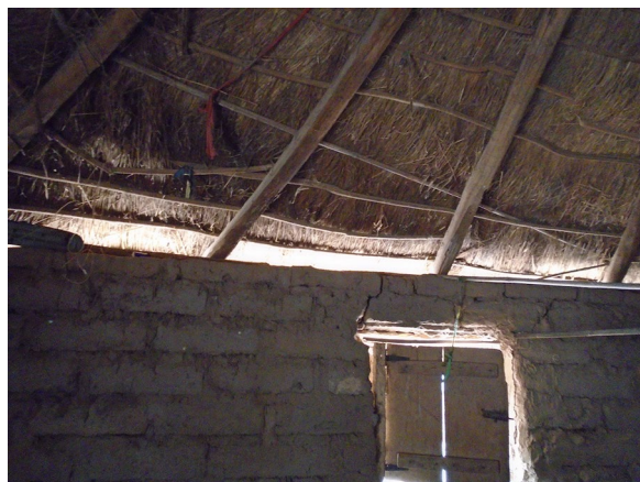
Fig. 7 PV Open eaves
