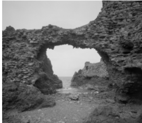
Figure 13.3 View of the covered passage leading from Dunbar Castle to the blockhouse.
