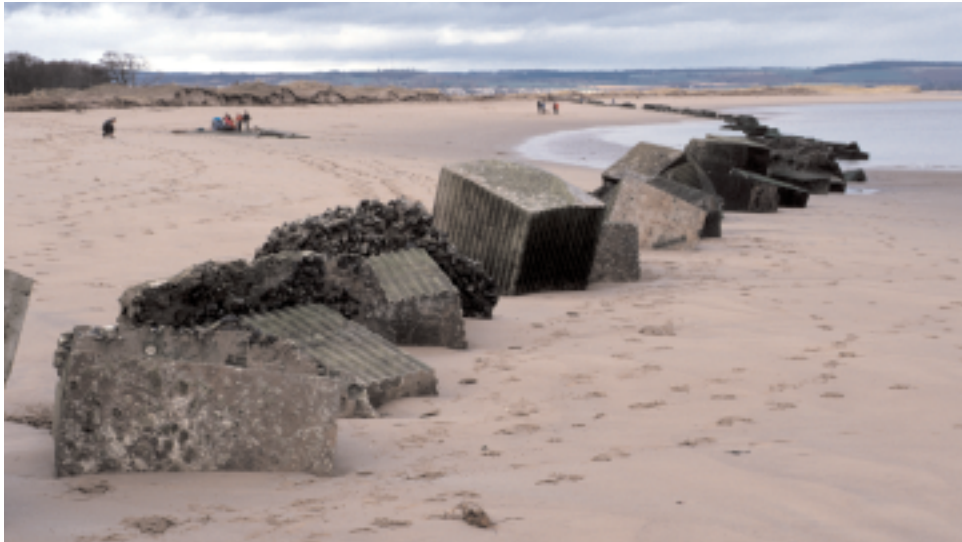
Figure 12.5. Collapsed tank traps at Tentsmuir; originally built on dry land.
