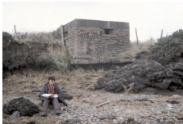
Figure 14.5. An eroding pillbox, one of many severely threatened sites from this period recorded during the survey.
