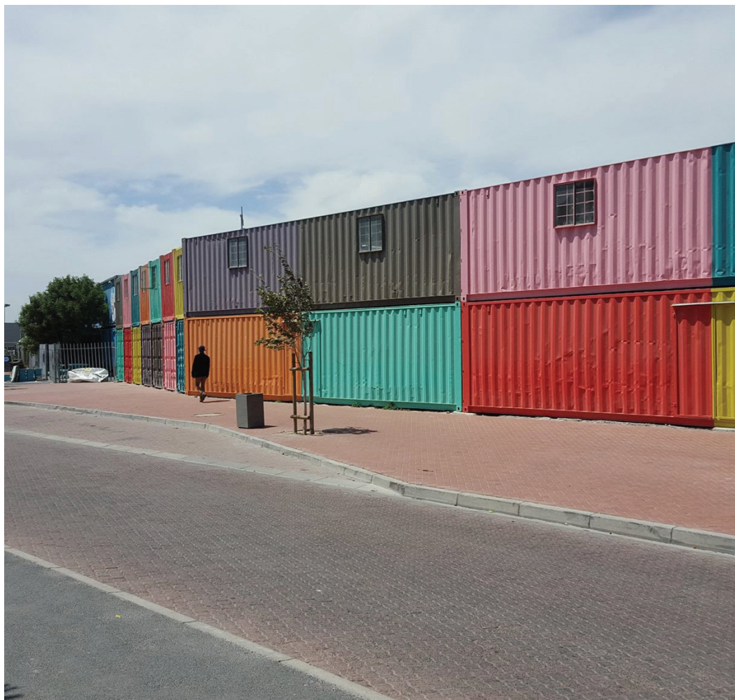
Image 12. The Container Walk, as seen from outside, and the refurbished footpath.
