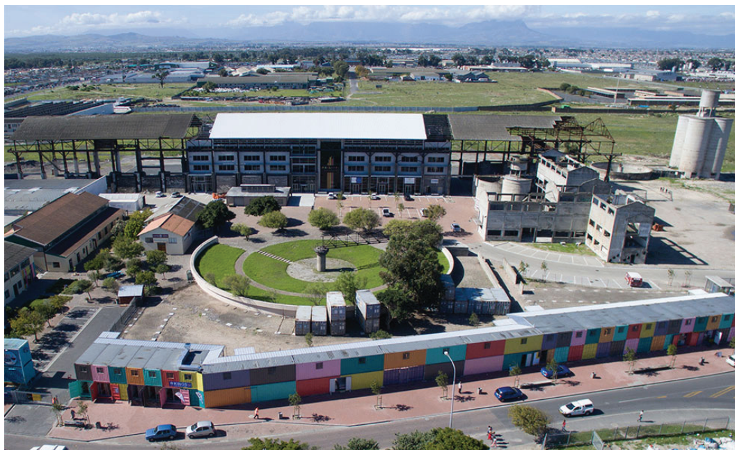
Image 13. A bird's eye view of the old cement factory now converted to office, workshop and retail space.
