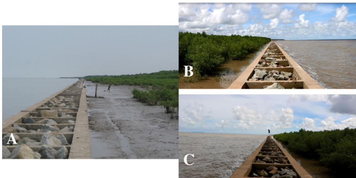
Figure 10. Incident waves at high tides did not overtop the HMS in November 2020, which was the period of highest tides in the area. (A) Low tide, and (B,C) high tides with strong incident waves.
