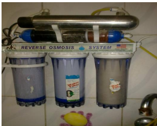
Fig.4: Reverse Osmosis system for drinking water used in current study.
