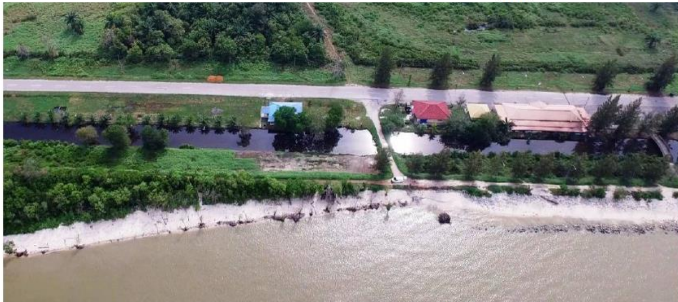
c) Aerial photograph of existing condition (20 th November 2015)
