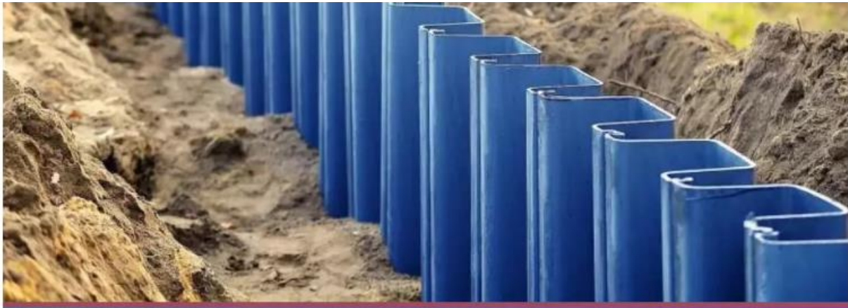
Figure 3.35 U-Type vinyl sheet piles
