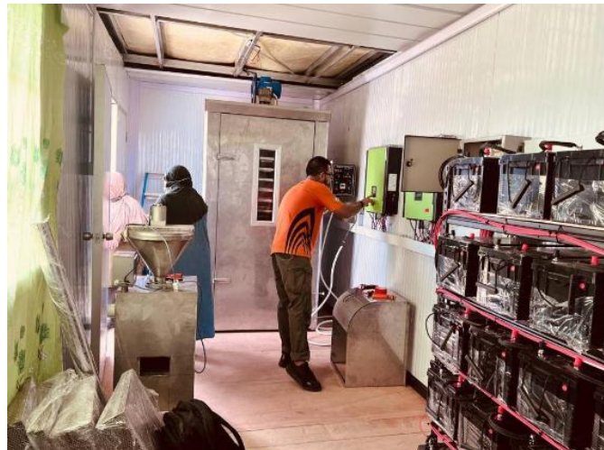
Gambarajah 9: Inverter Commissioning
