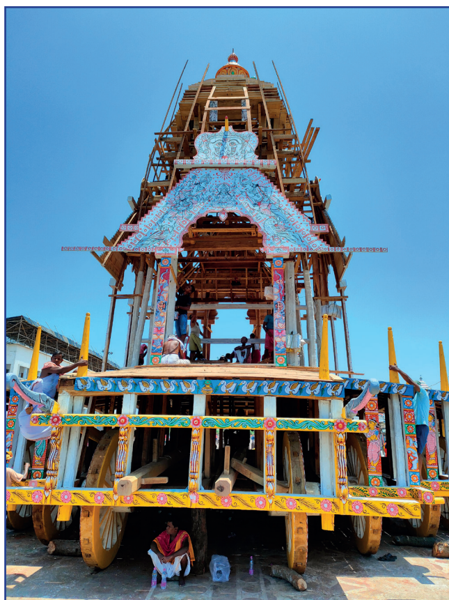
Figure 2: Chariot During Construction
