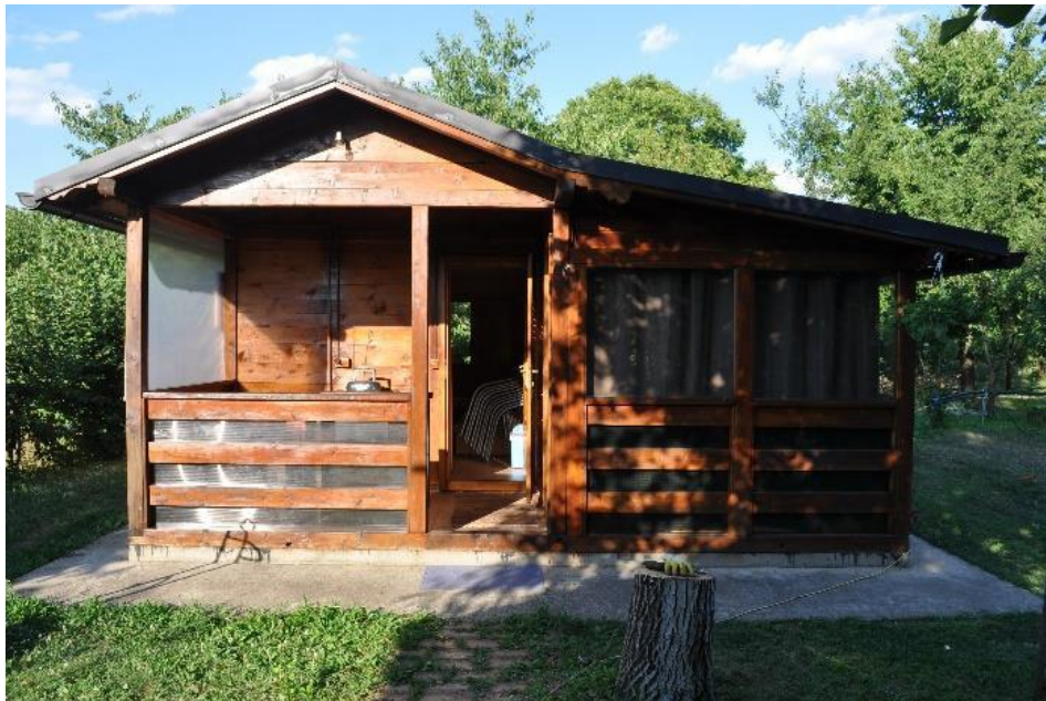
Figure 9. Summer cottage made of lightweight wooden boards used in the experiment.
