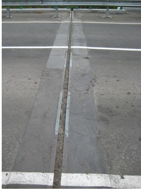
Fig. 1. Frame polymer concrete in expansion joint constructions.
