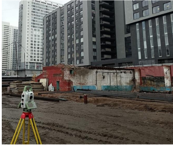
Fig. 2. Laser scanning of building structures scanning total station Leica MS60
