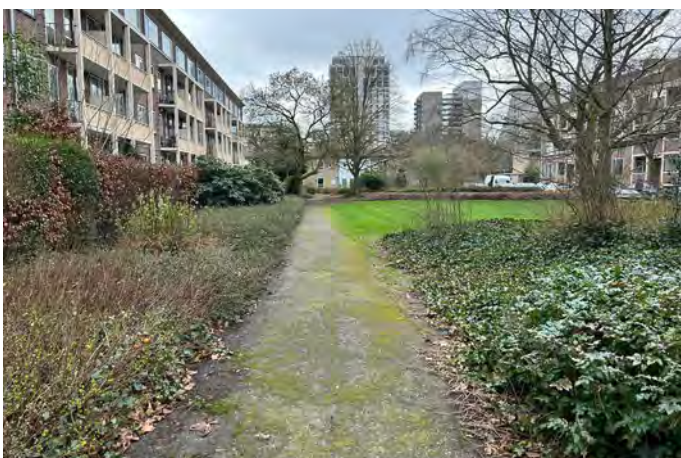
Image 39: Lack of maintenance (Limbeek Noord)
