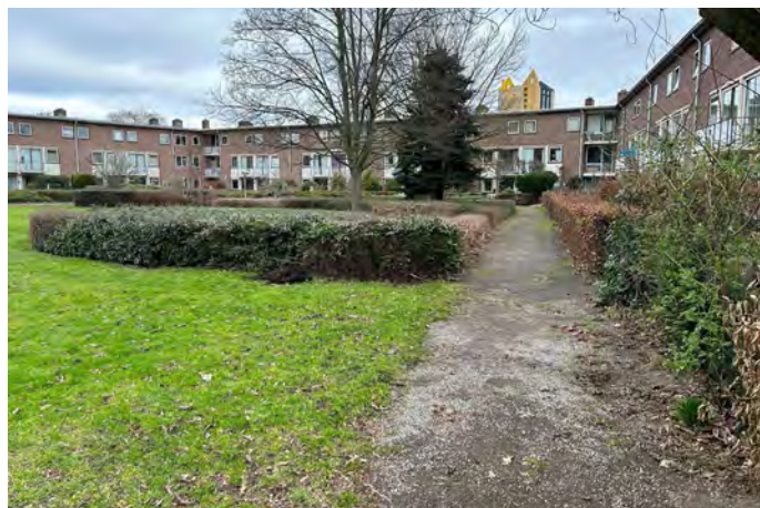
Image 40: Lack of maintenance in courtyards (Limbeek Noord)
