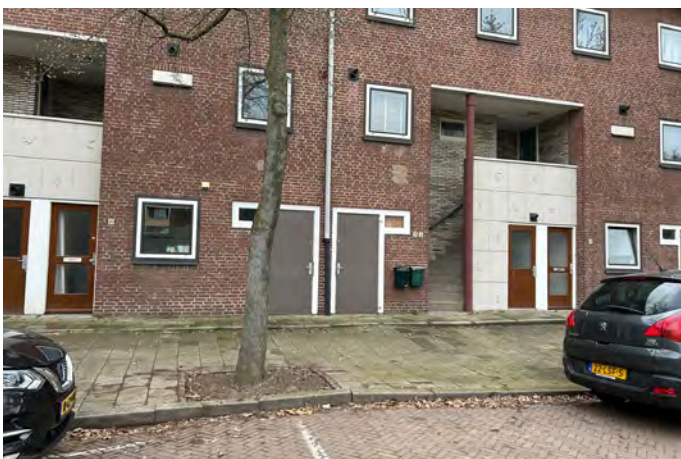
Image 37: Closed building facades (Limbeek Noord)
