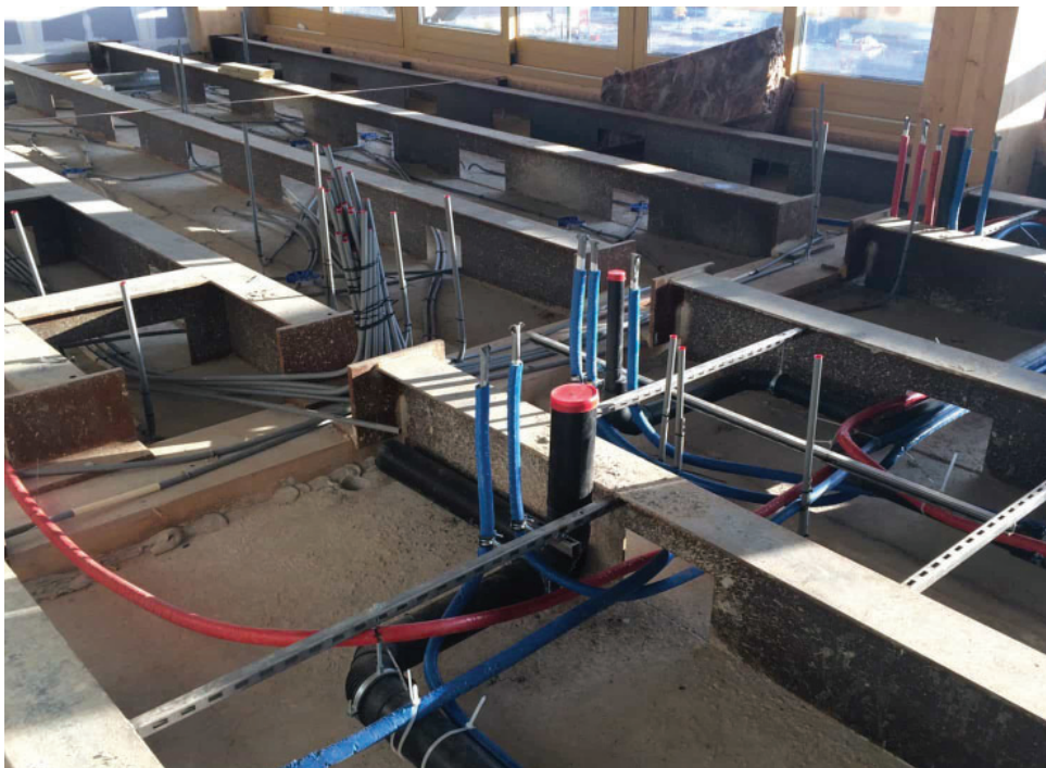
pipes in the floor, before the raised floor is finished
