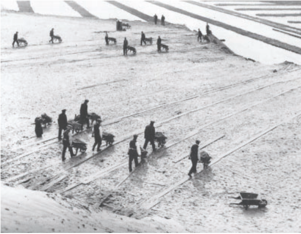
sand is poured for the new district
