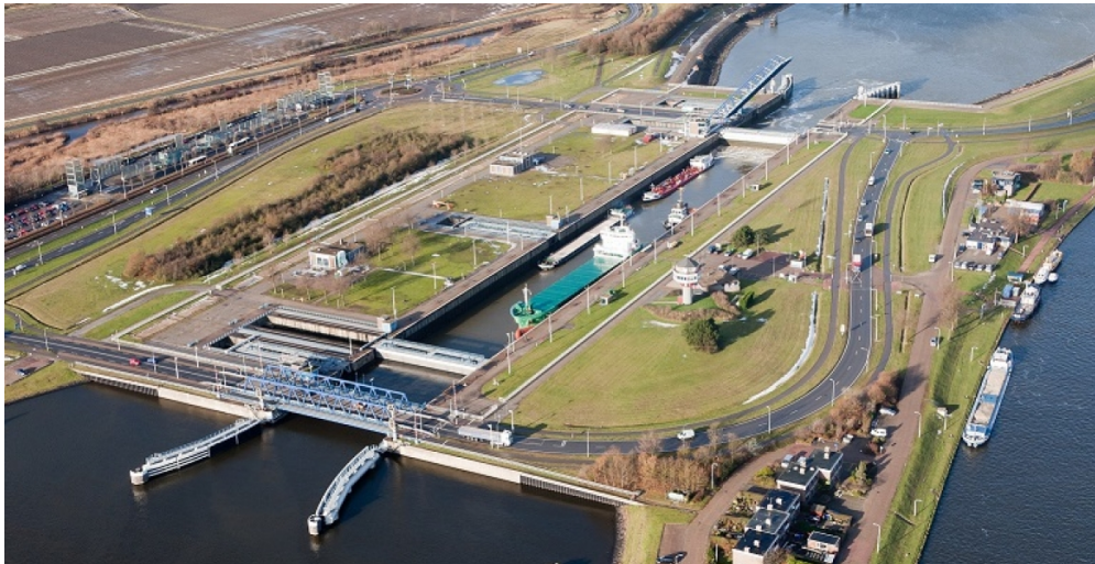
Figure 2: Westsluis located in Terneuzen. Image obtained from scheepvaartkrant.nl
