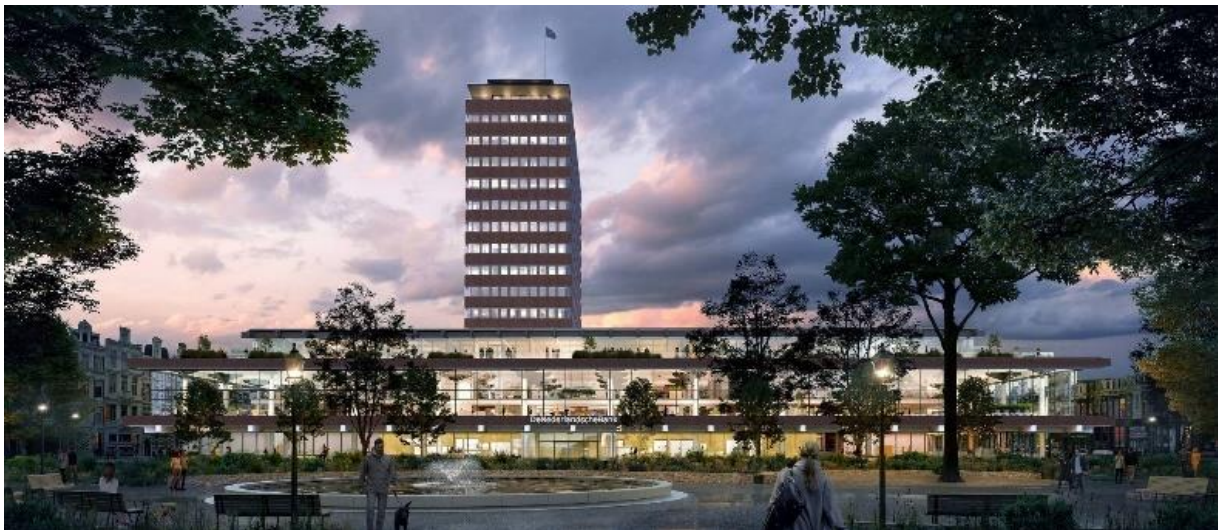
Figure 9: Renovation DNB with a modular construction (Strukton, 2021)
