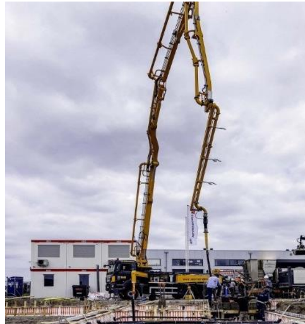
Figure 11: Circular concrete in foundation by new office Heembouw (Heembouw, 2021)
