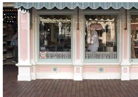
Figure 121. Hidden bakery air blowers (Photograph: Pinterest)
