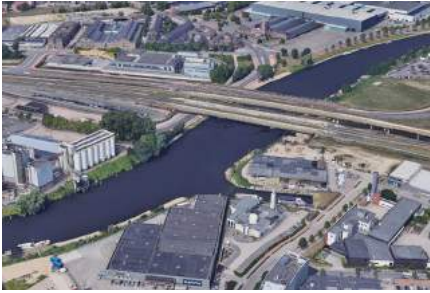
Figure 141. Railroad bridge (Photograph: GoogleEarth)
