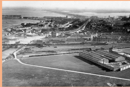
Figure 40. Aerial photo factory zone (Photograph: erfgoedshertogenbosch.nl)
