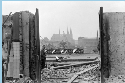
Figure 51. Demolishing of the industry (Photograph: erfgoedshertogenbosch.nl)
