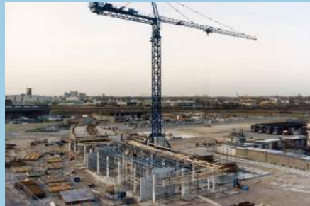
Figure 53. Construction police station (Photograph: erfgoedshertogenbosch.nl)
