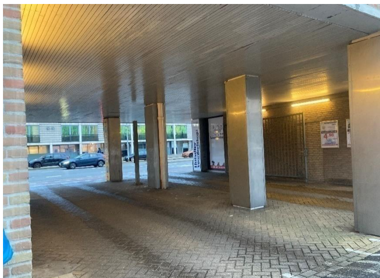
Figure 104: Carpark entrance from Boschdijk
