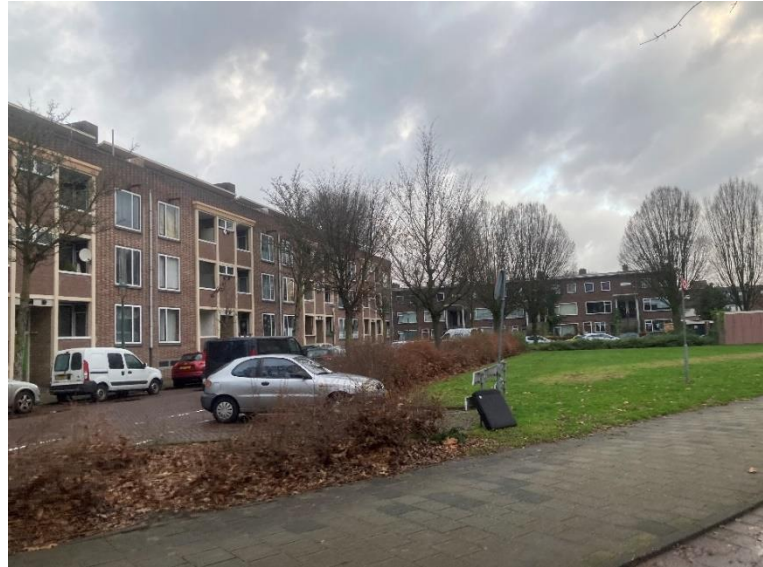
Figure 99: Portico flats at Steenstraat, Limbeek-North
