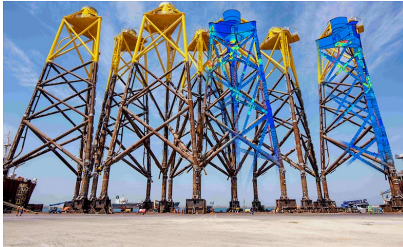
Figure 2.14: An impression of the steel structures for which the constructional physics and materials were tested using Akselos’ Digital Twin software [21]
