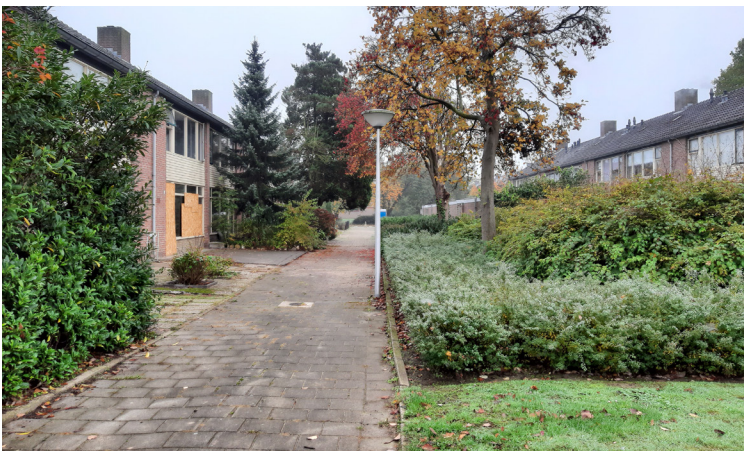
Image 32: unclear space between housing blocks in “strokenbouw”
