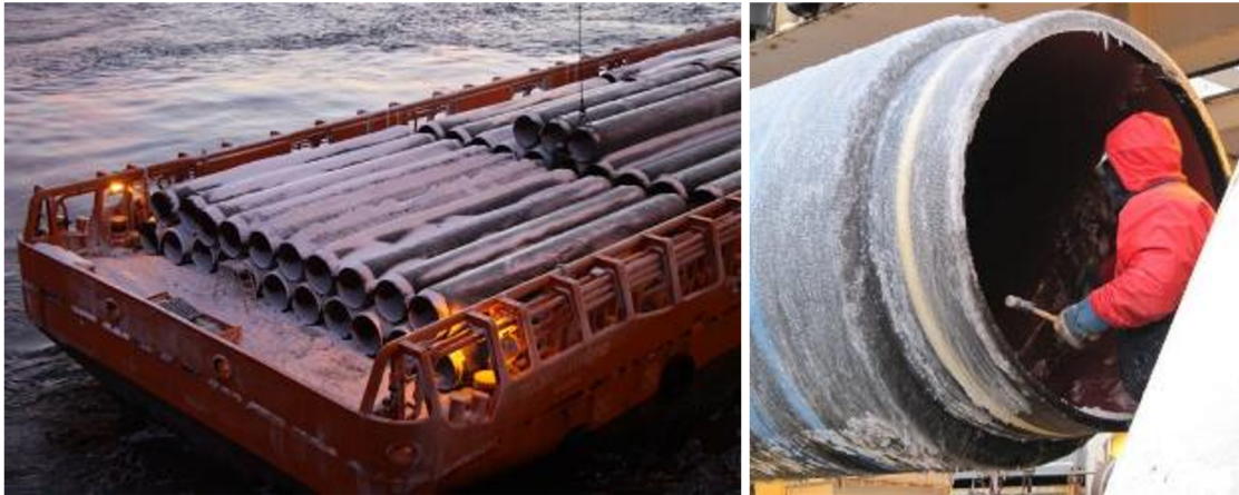
Figure 4.1: Ice accumulation on pipe joints [33]
