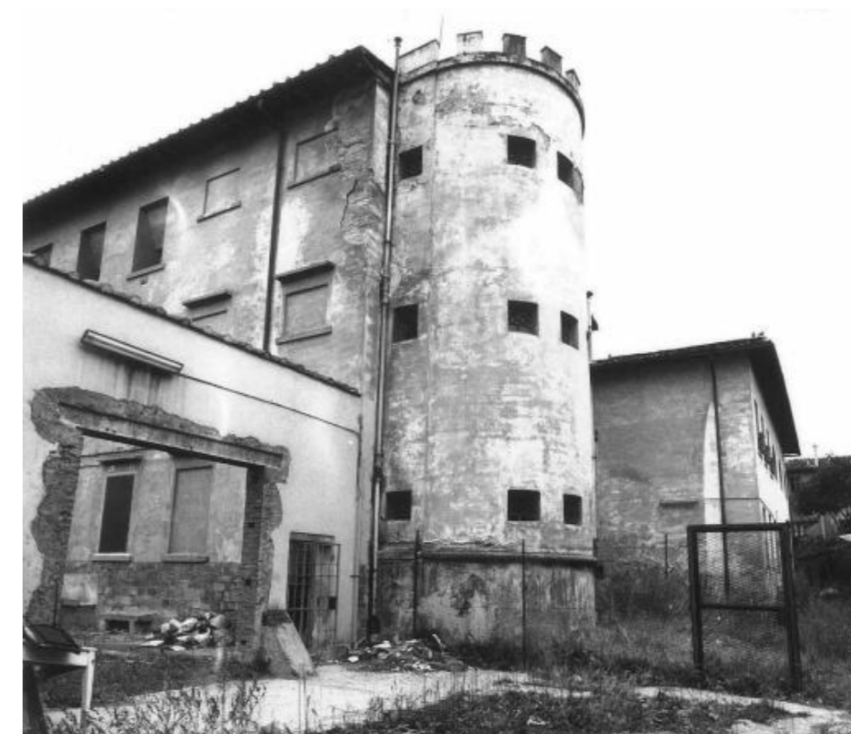
left 5-22 Connection space of the rooms used as general warehouses, 1984 right 5-23 First arm of the prison with a double order of galleries on east of structure, 1984 bottom 5-24 Prison branches on east of structure
