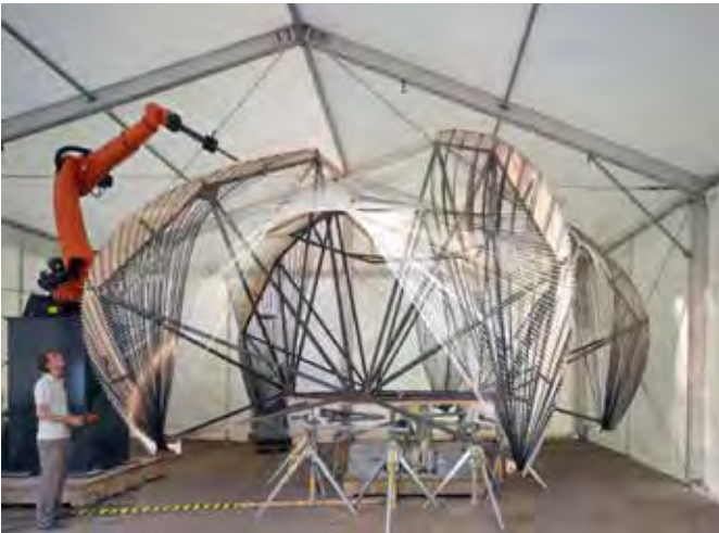
Figure 38 (ICD / ITKE University of Stuttgart, 2012) The setup for assembly with a 6-axis Kuka robot
