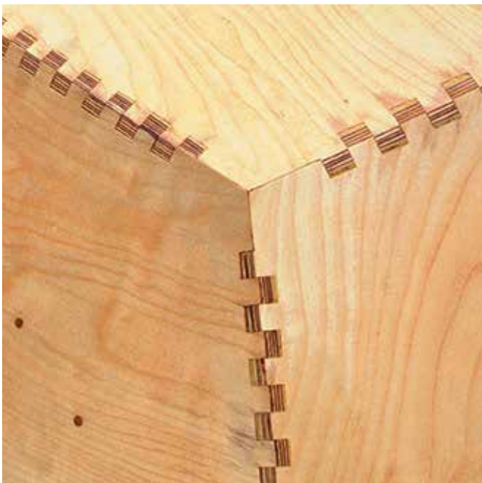
Figure 23 (ICD / ITKE University of Stuttgart, Roland Halbe 2011) Finger joints connecting the plate.
