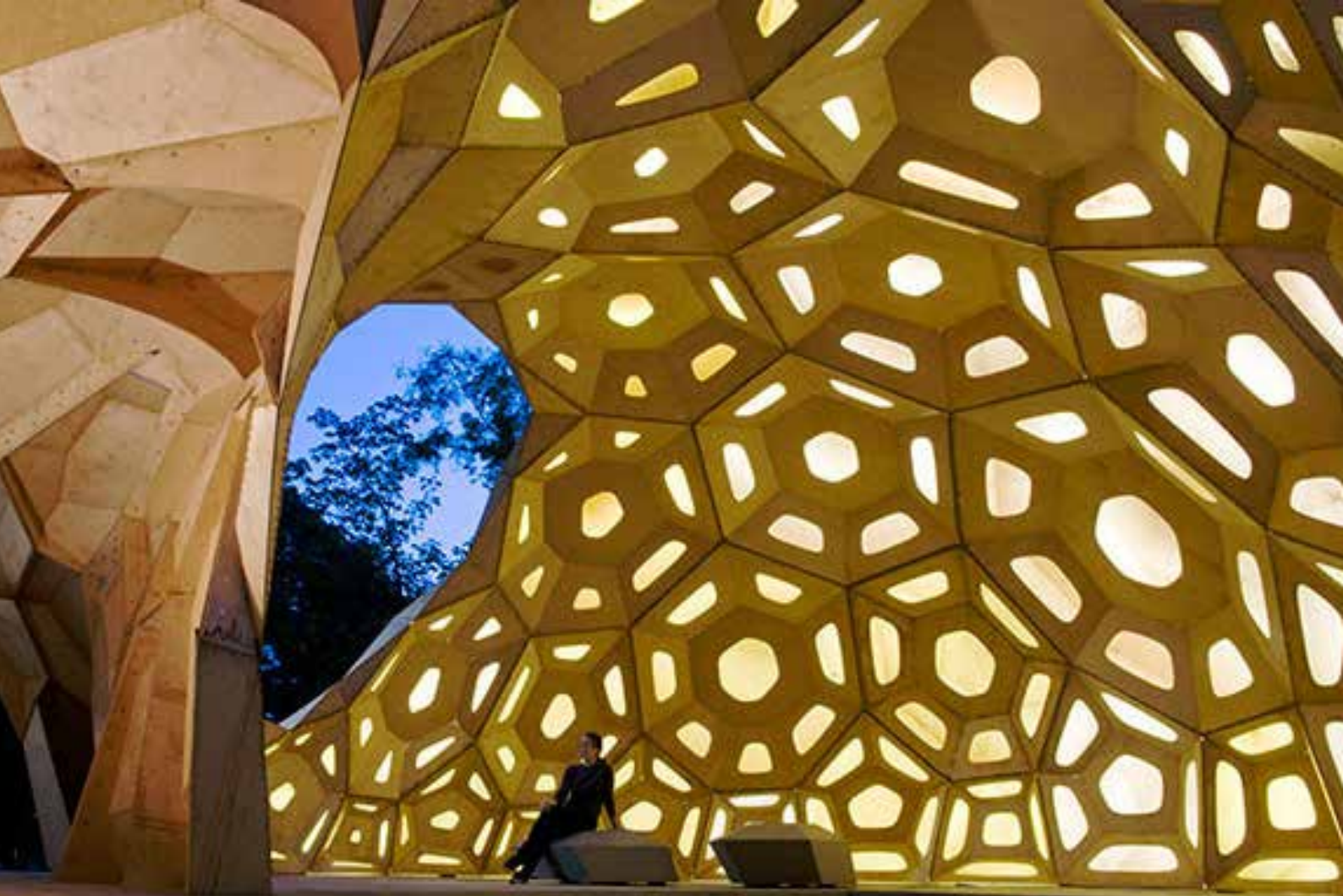
Figure 10 (ICD / ITKE University of Stuttgart, Roland Halbe, 2011) Research Pavilion 2011 Photo of the actualized pavilion.
