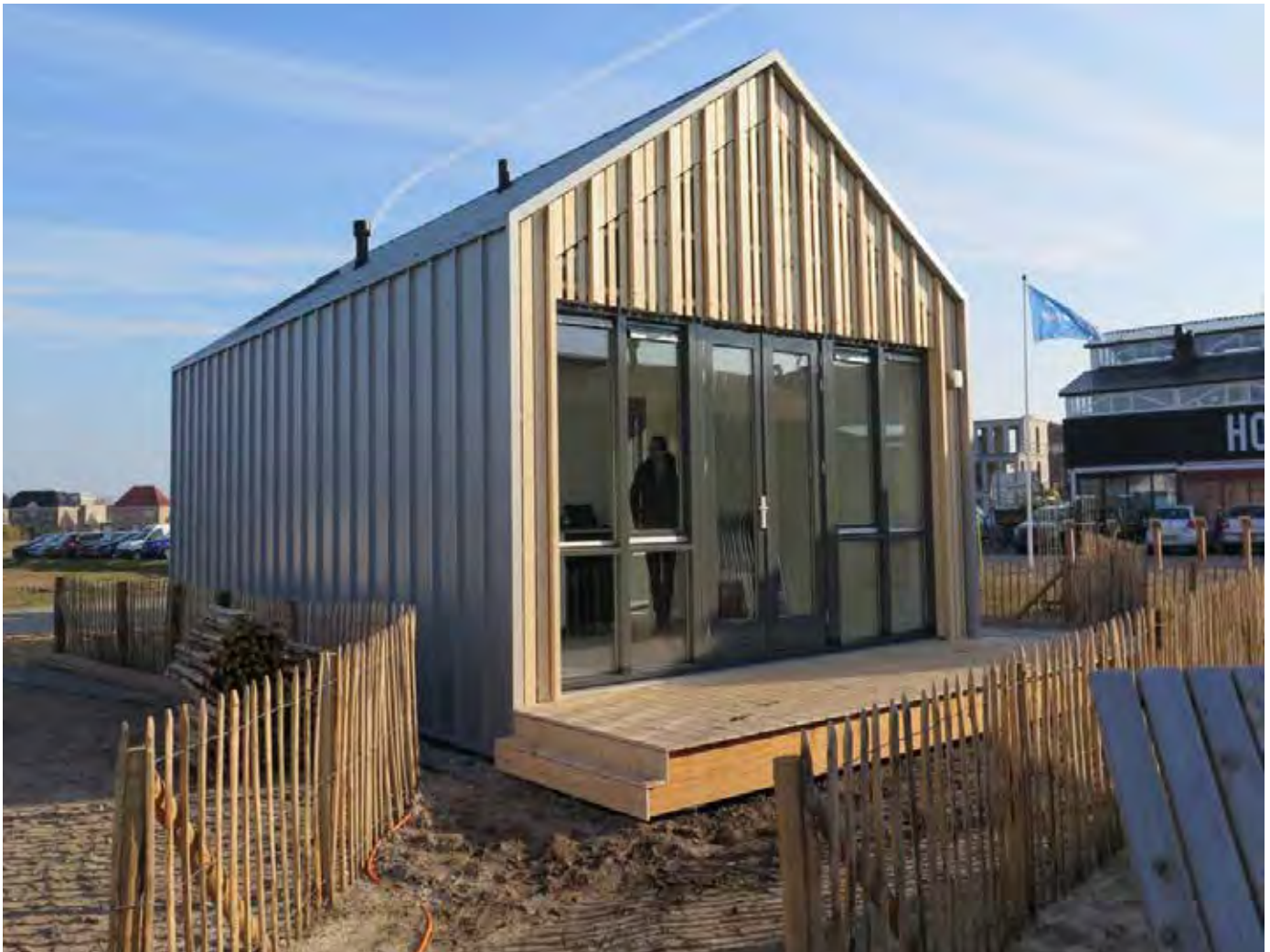
A.13 a finished WikiHouse in Almere, the Netherlands (Keratoop, n.d.)
