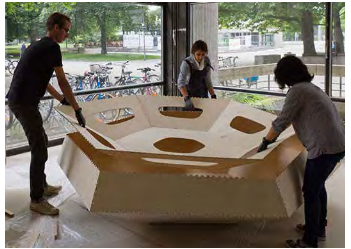
Figure 20 (ICD / ITKE University of Stuttgart, Roland Halbe, 2011) Assembling plate cell made of plysheets.
