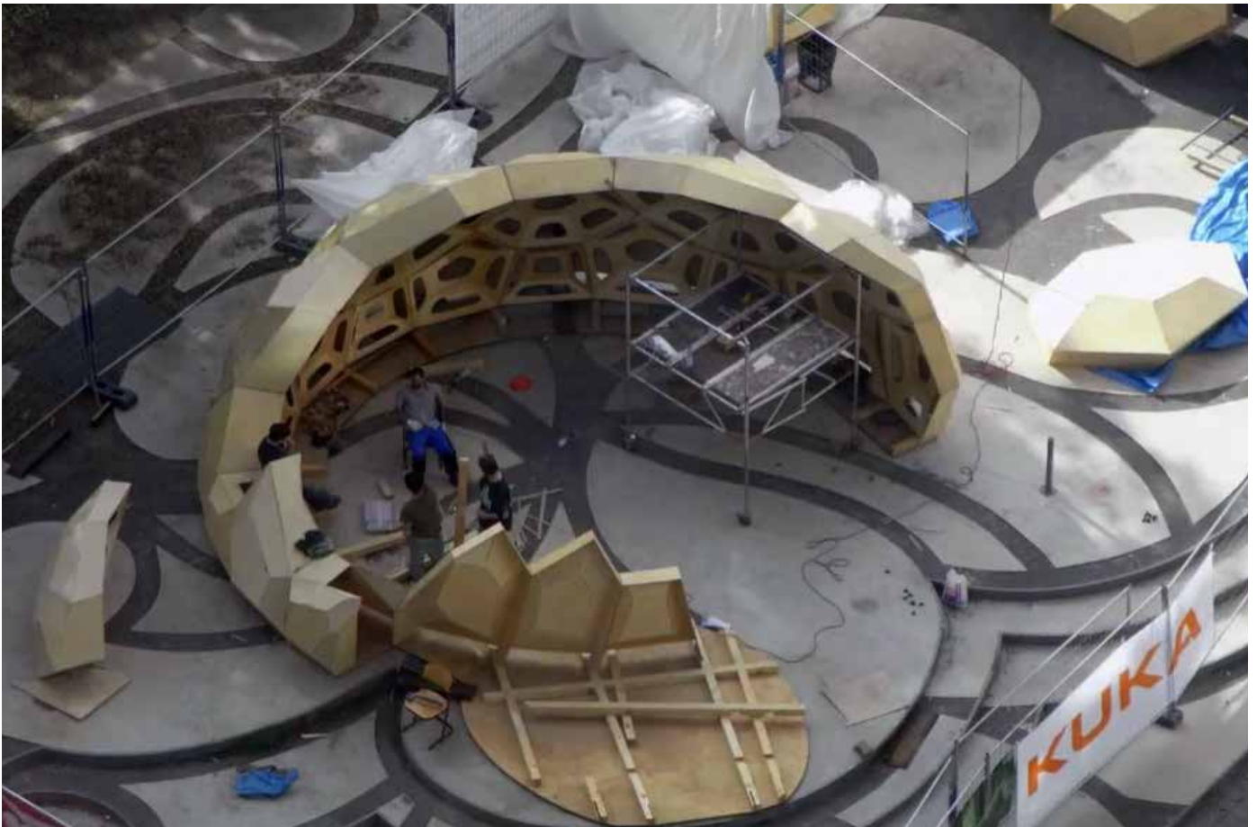
Figure 27 (ICD / ITKE University of Stuttgart, 2011) Assembling process on site-Step 1.
