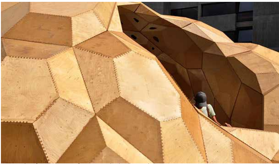
Figure 11 (ICD / ITKE University of Stuttgart, Roland Halbe, 2011) Close image of the plate structures inspired by the sea urchin.
