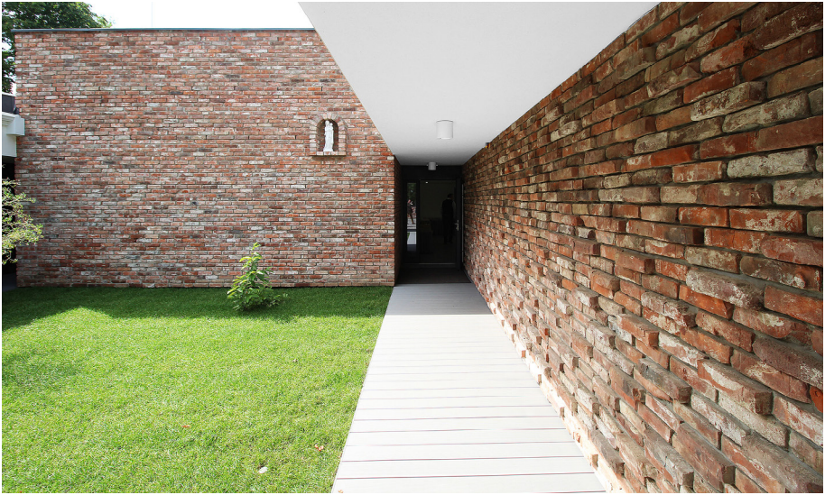
Fig. 2.4.1.2 Recycled brickwork in the facade [One Light Studio, n.d.]
