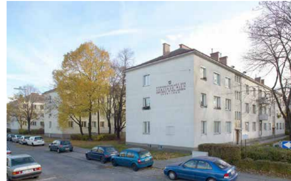
Figure 3.6 Post-war social housing estate on Wagramer Straße 164-168 in Vienna (Stadt Wien, n.d.)
