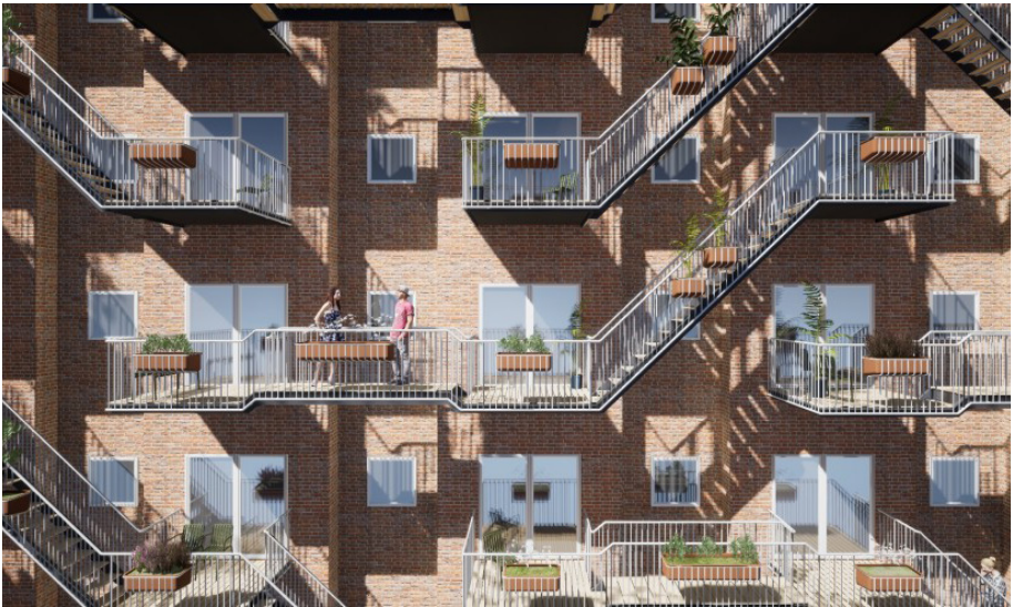
Fig.2.2.3.3 Facade [Van Capelleveen, E., n.d.]
