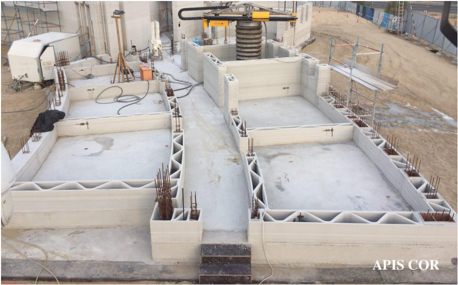
Fig. 3.5.2.3 concrete printed walls with steel rebars [Harrouk, C., n.d.]
