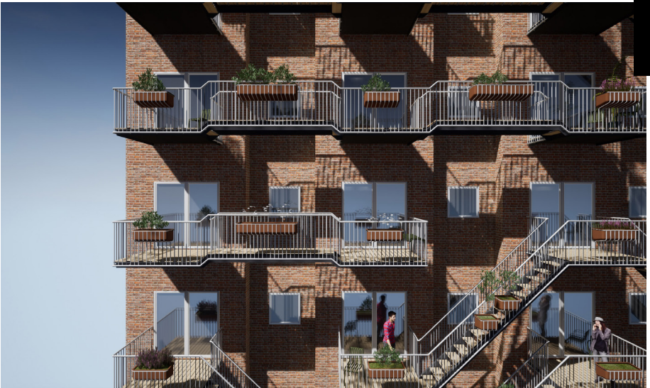
Fig. 2.2.3.5 Facade [Van Capelleveen, E., n.d.]
