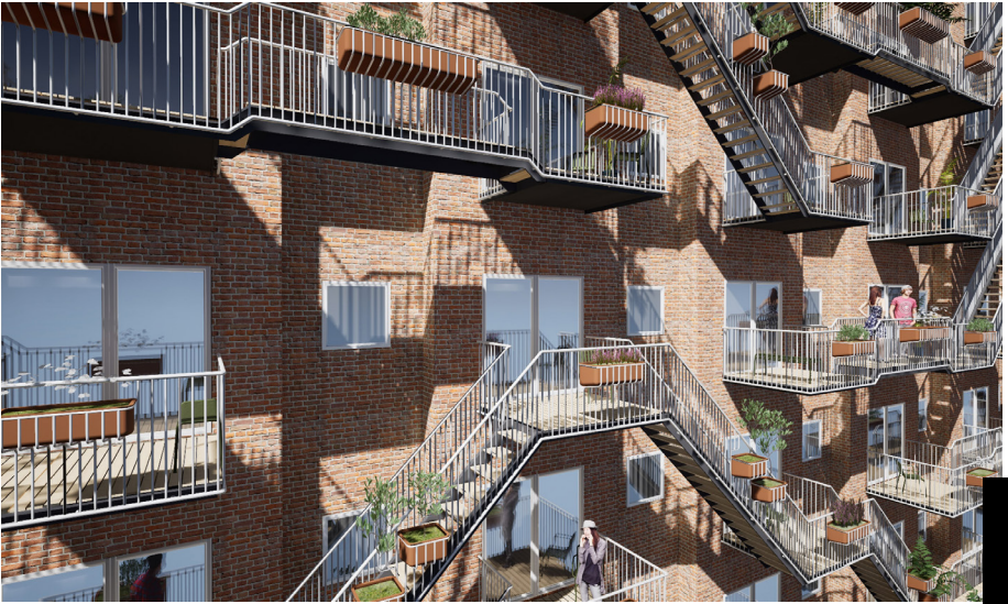
Fig. 2.2.3.4 Facade [Van Capelleveen, E., n.d.]
