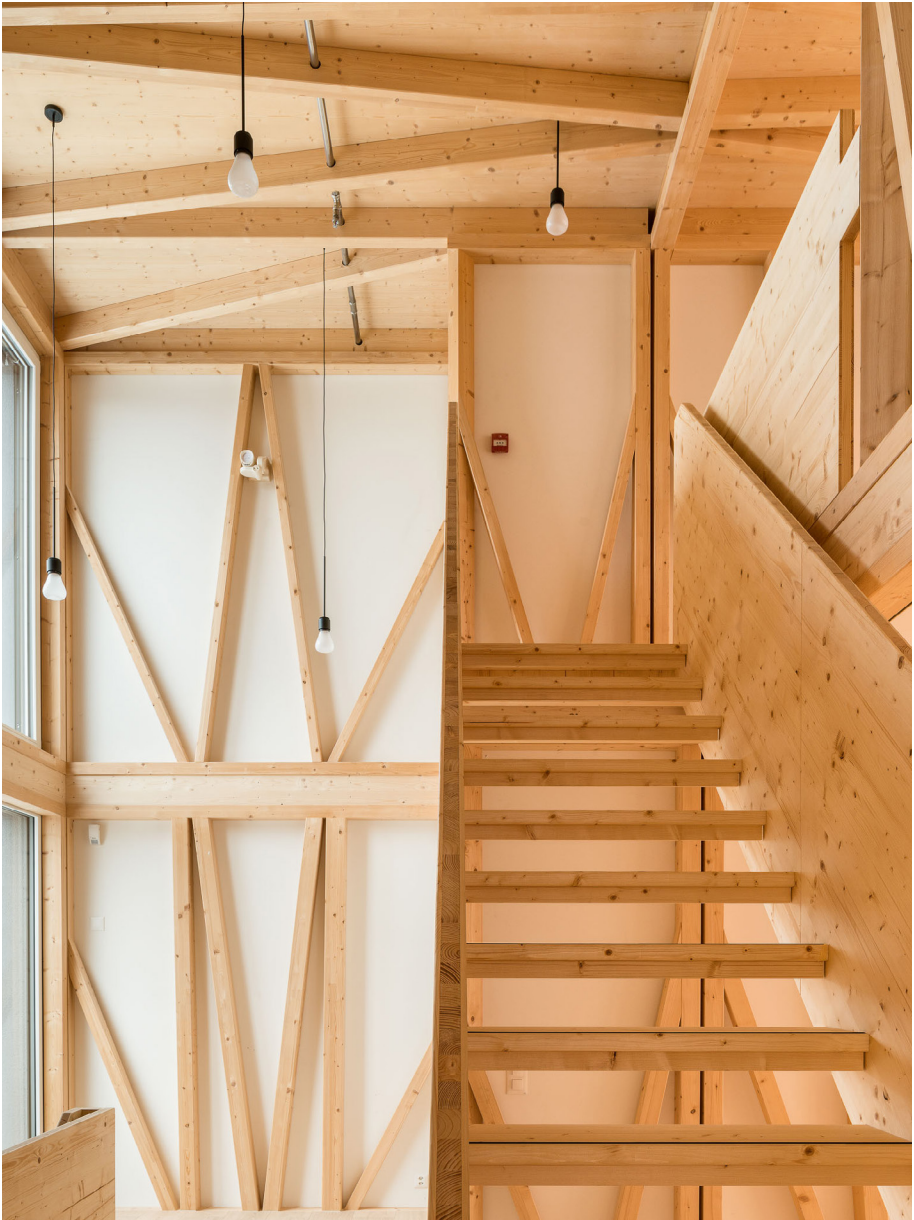
Fig. 3.5.5.8 The wooden structure [Mac, D., n.d.]
