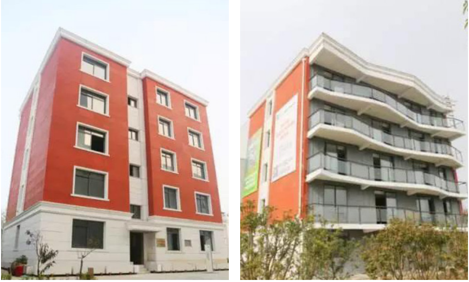
Fig. 3.5.4.2 First 3D printed project by Winsun3D [Winsun3D, n.d]
