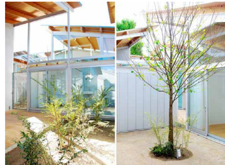
Figure 5.2 Inner gardens of the Nishinoyama House (SANAA Architects, 2016)
