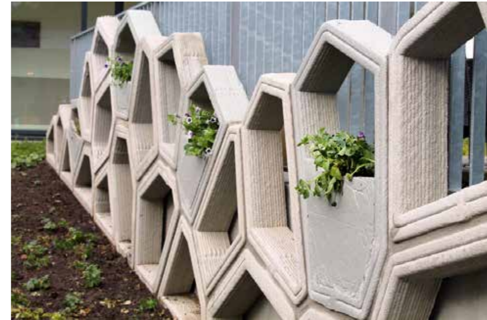
Figure 2.08 Voronoi 3D concrete printed wall (Vertico, Saxion Industrial Design Research Group, De Witte van der Heijden Architecten, & Trebbe, 2016)
