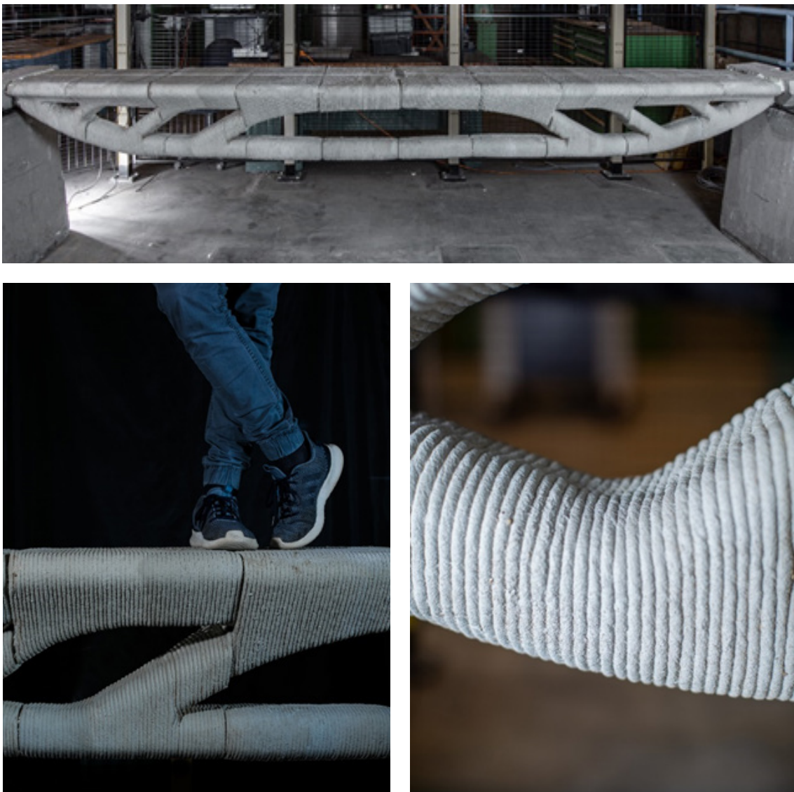
Fig 4.4: Topology optimized bridge by the University of Ghent [54]
