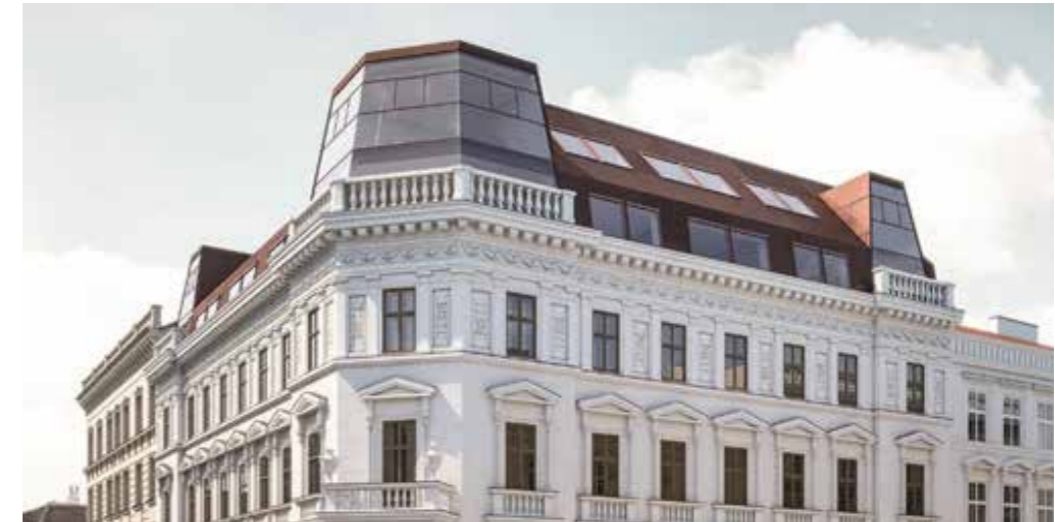
Figure 3.5 Attic extension on an 19th century building in Vienna (HMA, 2017)
