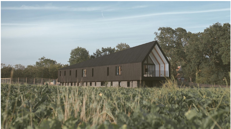
The offgrid Black Barn produces self-sufficient energy. [Crook, L., 2019]
