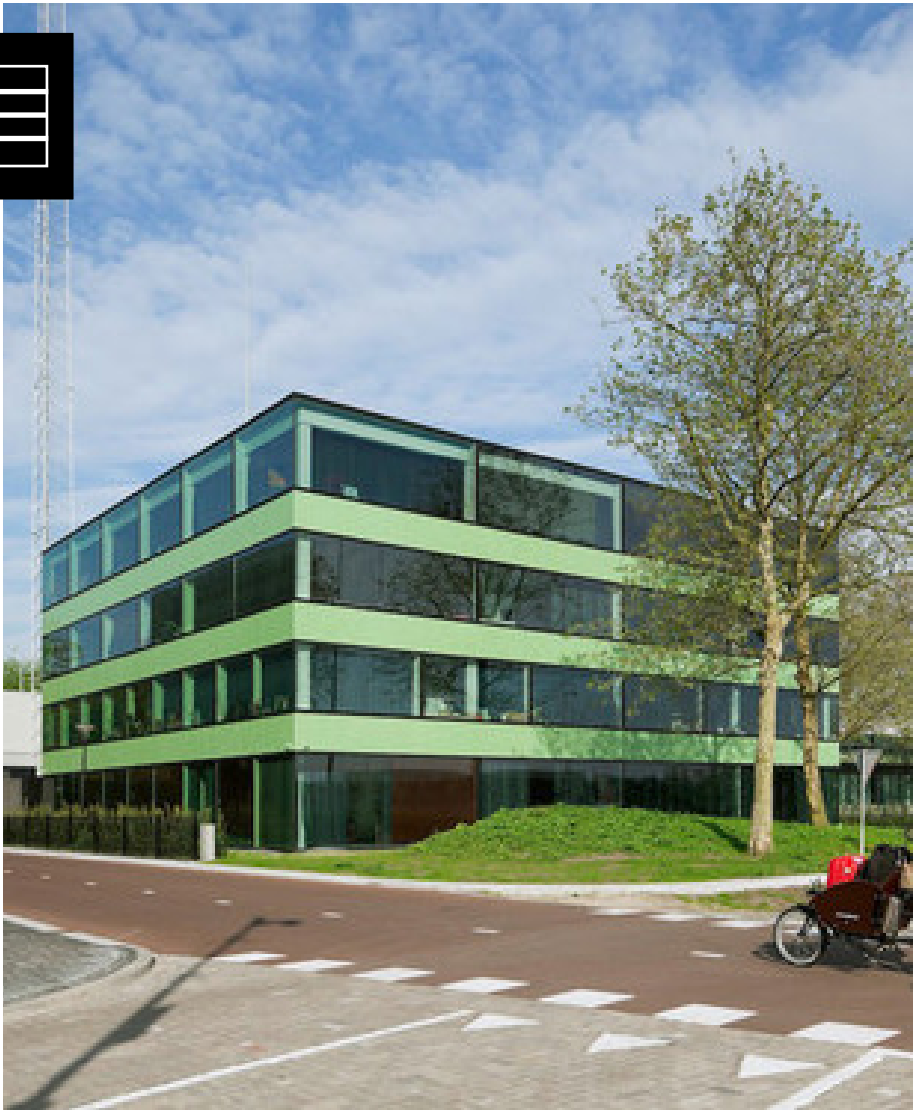
Fig. 2.3.2.1 Exterior [Archdaily,, n.d.]
