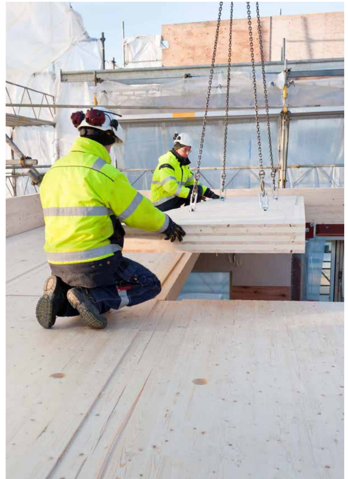
Figure 5.6 Mounting of CLT panels (RISE Research Institutes of Sweden, 2019)
