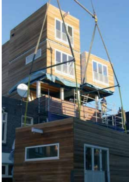
Figure 3.2 Hoisting the housing units on new construction (DAAD Architecten, 2005)
