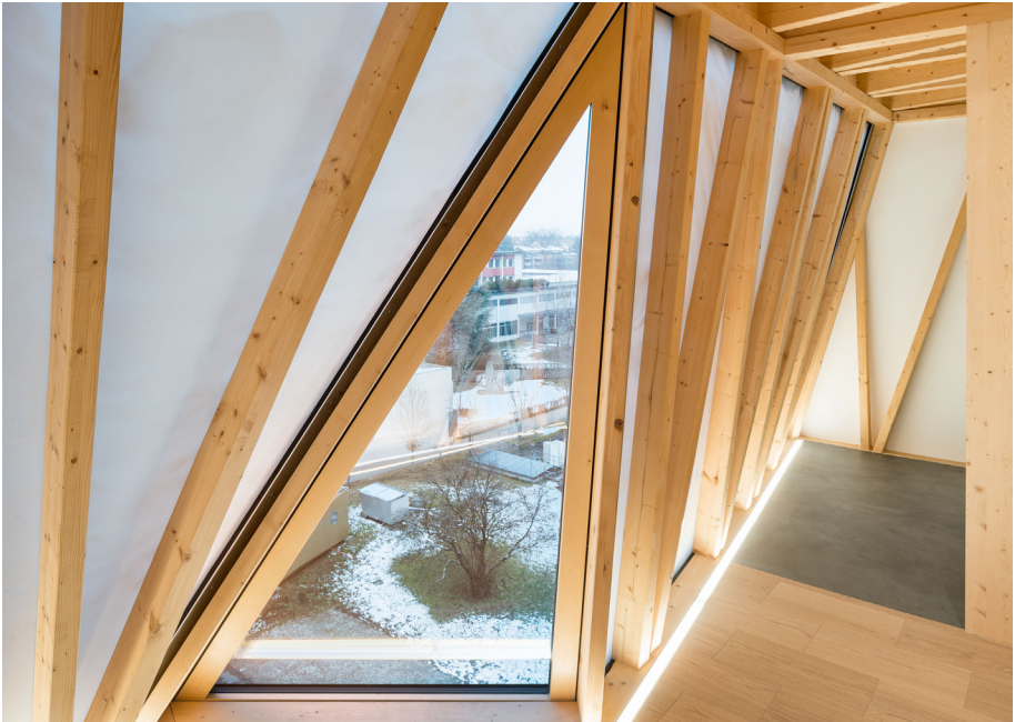
Fig. 3.5.5.9 wooden structure with double layered membrane [Mac, D., n.d.]
