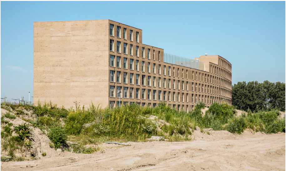
Fig. 1.4.1.4 Back of the building [Cuypers, P, n.d.]
