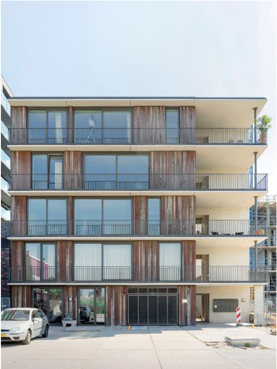
Fig. 3.2.1.2 Front of the building [GAAWAA, n.d.]
