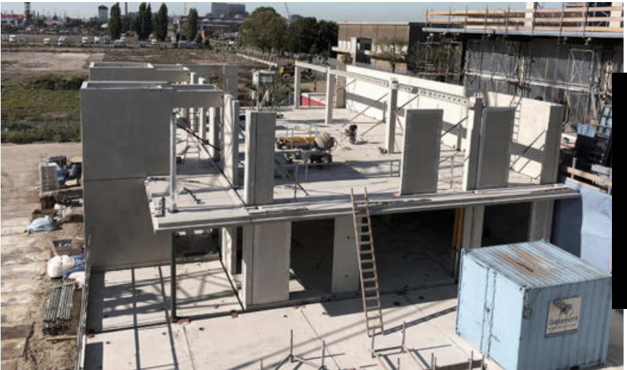
Fig. 3.2.1.4 Construction site [GAAWAA, n.d.]
