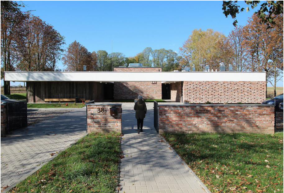
Fig. 2.4.1.1 Front facade of the shelter [One Light Studio, n.d.]
