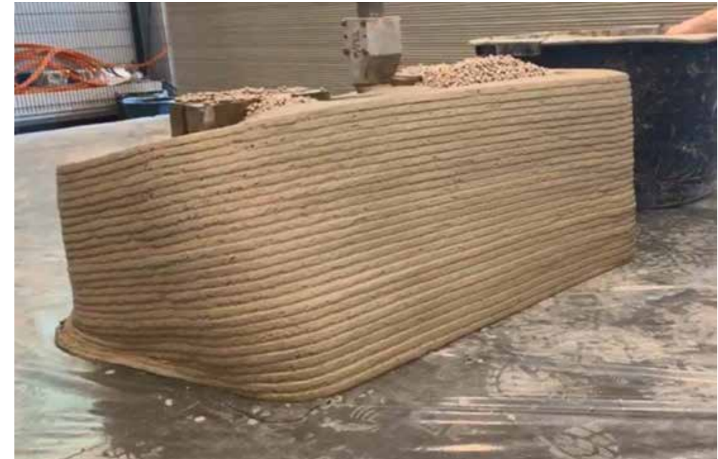
Figure 2.06 Buckling of 3D printed concrete structure due to inappropriate buildability (photographed at TU/e)
