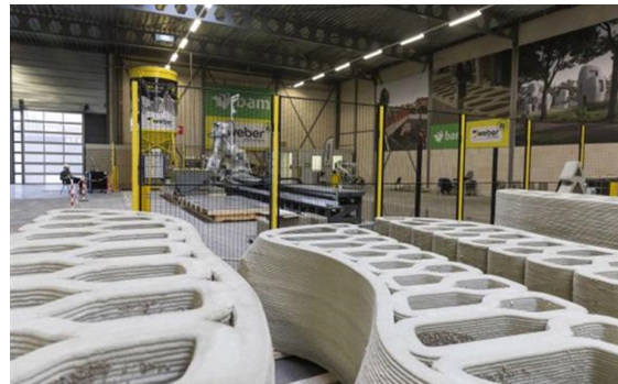
Fig 4.10: 3DCP cycle bridge elements in the Netherlands
